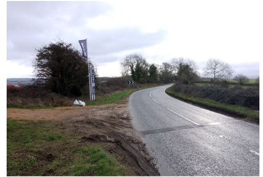
Dangerous bend on the Oddington Road
